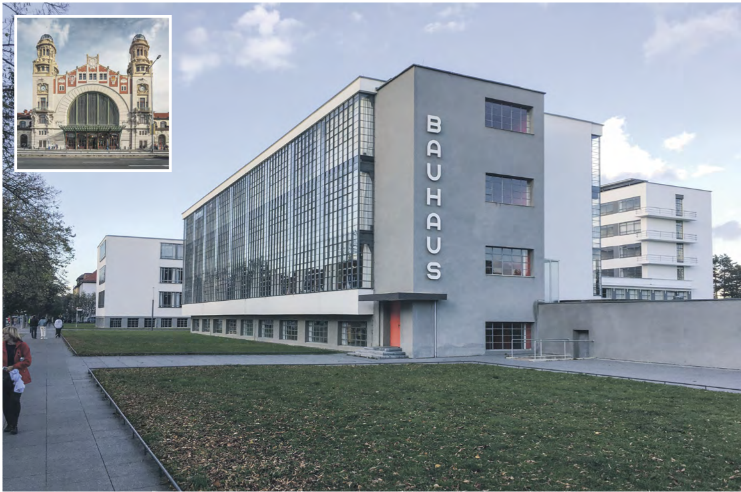
Budova školy Bauhaus, Dessau | Bauhaus Building (1925-26)
